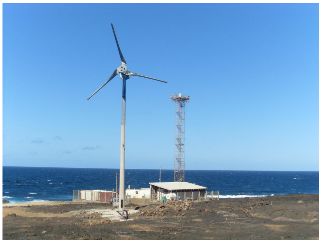
Figure 1. The CVAO complete with newly erected wind turbine.
