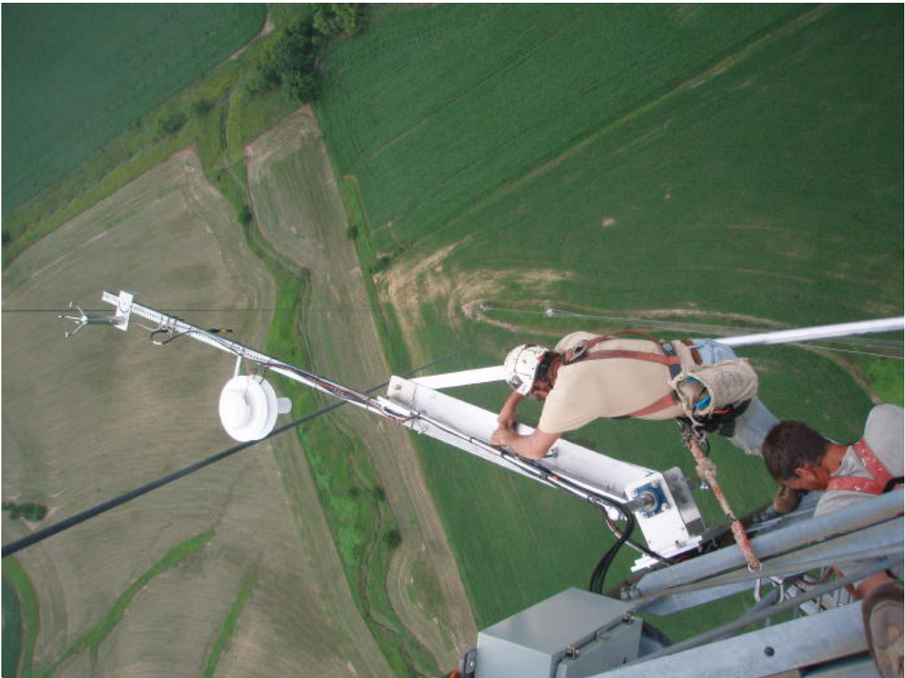
Figure 1. Air Intake at West Branch Iowa Tower
